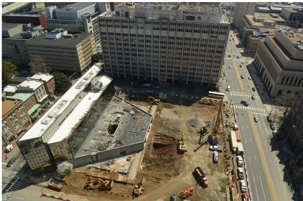
Figure 2. Existing Building Prior to Demolition (credit Elmquist)
