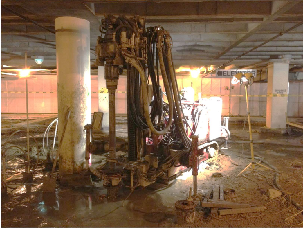
Figure 9. Micropile Installation
